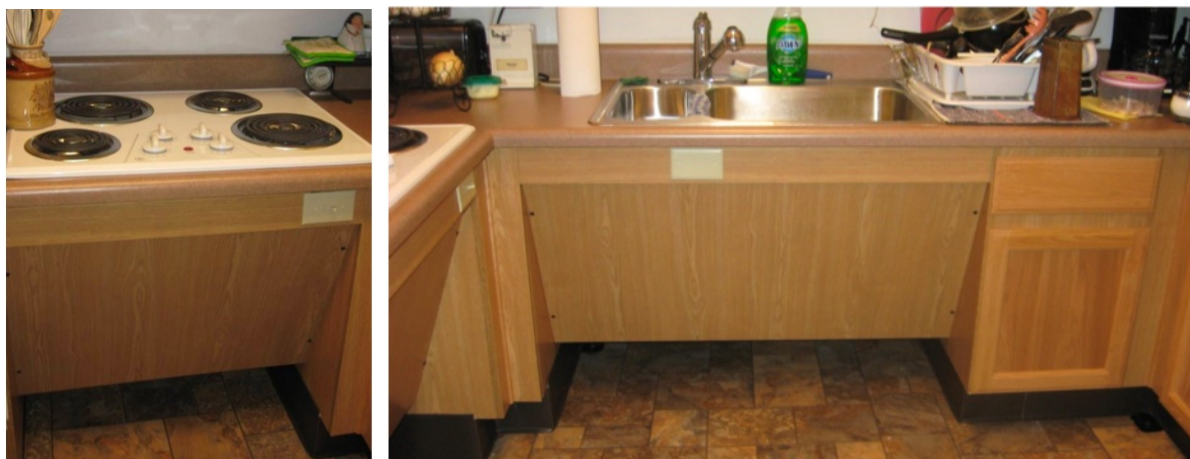
Figure 4 and Figure 5 Kitchen in ADA-Designated Units
